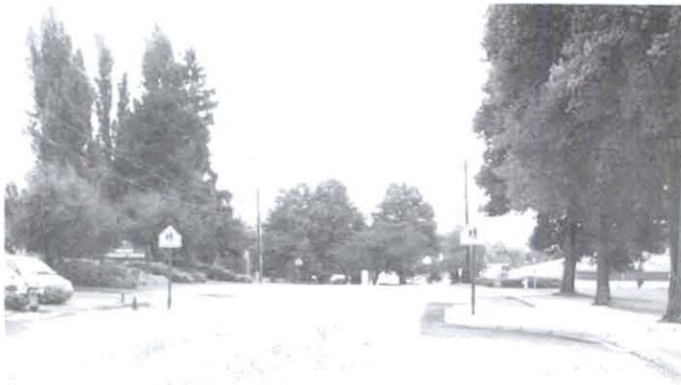
The project within the school zone in front of Midway Intermediate School and Pacific Middle School included the construction of a widened sidewalk at the school crosswalk and improved signage.
